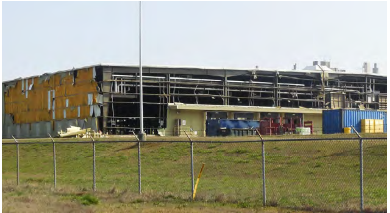
Closure of the International Paper plant in Courtland left about 1,100 workers without jobs. [Michael Wetzel/Decatur Daily]
