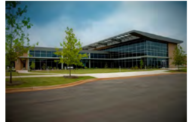
One of the RTP training facilities.
